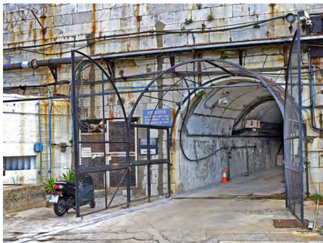
The Admiralty Tunnel Dockyard portal
